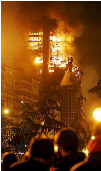
Der Windsor Tower in Madrid, 2005
